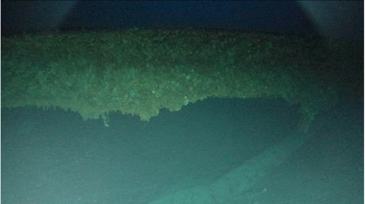
This continues to show the damage on the port side of Yamashiro's engine room. Her entire port side is open to the sea. ( Yamashiro's engine spaces occupied roughly frames 190- 224) (Photograph provided by Lone Wolf Media. )
