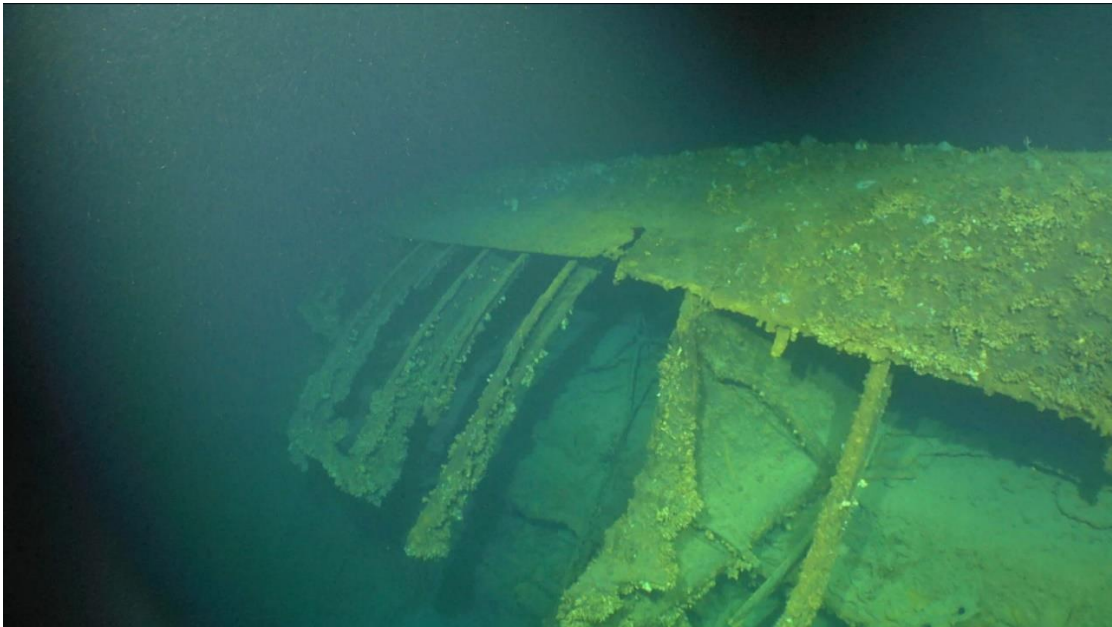
This is moving forward on Fuso approximately frame 210 on her port side showing that this area is devastated. The area of damage is so great that it is very likely it was caused by two torpedoes striking her in close proximity to each other. (Photograph provided by Lone Wolf Media.)
